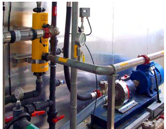
RO recovery device.
